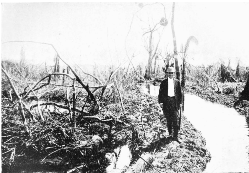
Figure 10.5 Jungle trees killed by the “hydraulic fill” on the west bank of the French Canal at Gatun. From the swamp created by the fill enormous swarms of Anopheles flew to Gatun, which is over a mile from the swamp.
