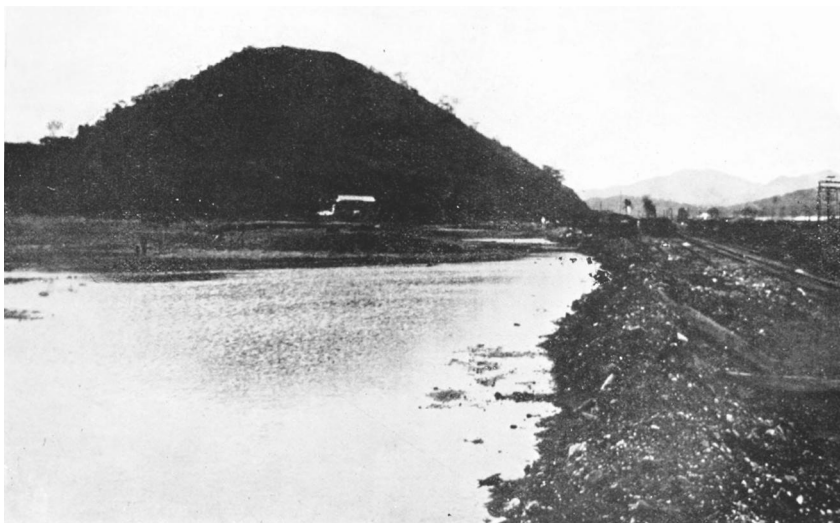
Figure 10.3 The “hydraulic fill” at Balboa. The future site of the official quarters of the Port of Balboa, at the Pacific end of the Canal. Originally a mangrove swamp, the ground level is being raised by pumping liquid mud onto it. The large pipe discharging the mud is seen in the middle of the swamp. The hill in the background is Sosa Hill. On the right of the railway the new docks are being constructed, and it is from them the mud is being pumped to raise the site for the new port.
