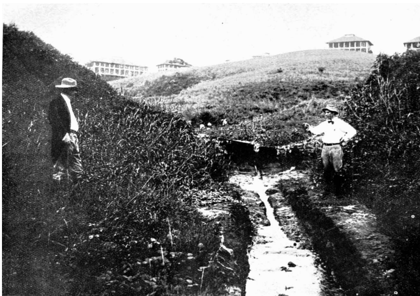
Figure 11.1 Tile drains ending in an open drain cut in rock, at Gatun, Panama. Men seen in the middle distance of the photograph are relaying the pipes, which had been blocked by grass roots.
