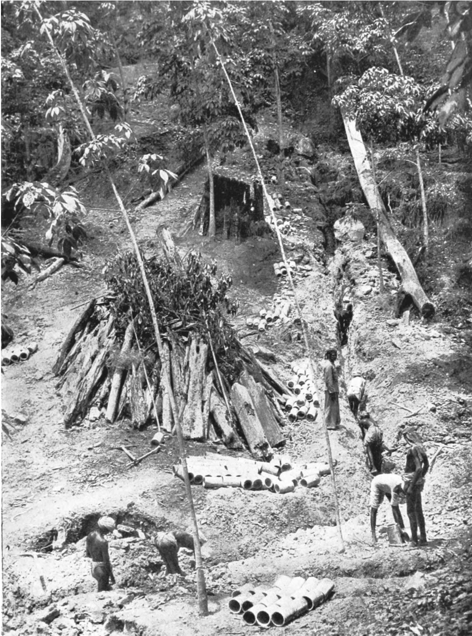
Figure 2.3 Bukit Ijok estate, Federated Malay States. Subsoil drainage to tap springs on the side of a steep ravine.
