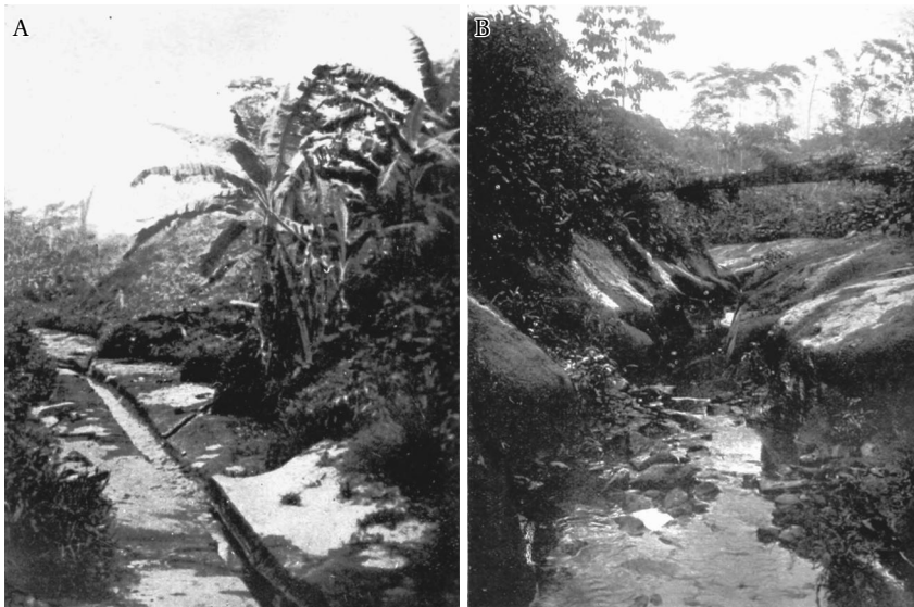
Figure 10.8 Ravines at Gatun, before and after drainage. A: an open drain has been cut in the soft sandstone of this ravine. B: a branch of the same ravine which has not been dealt with by the Sanitary Department.
