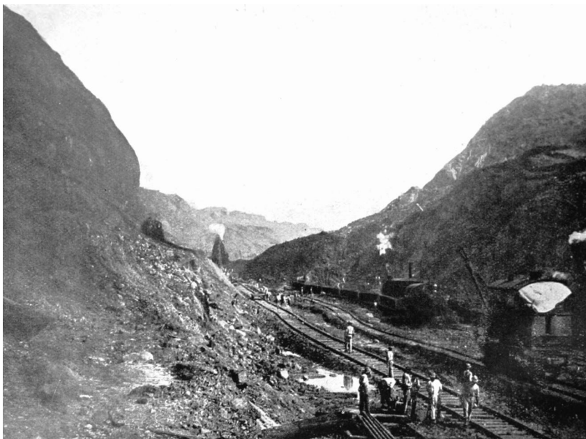
Figure 10.18 The Cucaracha slide on the right is seen blocking the Cut, which has been cut through to the bottom level a few days before. Above the slide is Gold Hill. The houses on the right edge of the Cut in the distance are at Culebra. At this point the Cut is nearly 500 feet deep, of which 300 feet have been excavated.
