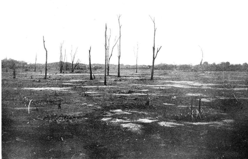
Figure 10.6 Land raised by hydraulic filling on the east bank of the French Canal at Gatun. The remains of the swamp trees are still to be seen.
