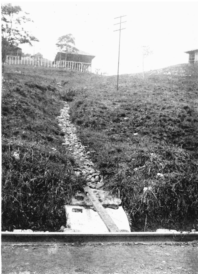
Figure 10.2 A Subsoil Drain covered by stones at Ancon. To prevent water from the pipe washing away the railway line, the end of the pipe discharges below and against a concrete covering.
