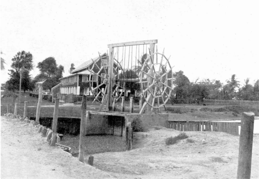
Figure 17.2 British Guiana: A “koker,” or hand-worked tide gate
