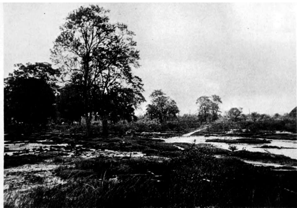
FIG. 35.—ON THE EAST SIDE OF THE ROAD FROM COLON TO MOUNT HOPE. The land is very swampy, being covered by all tides. The photo shows one of the shallow drains employed to drain this almost undrainable swamp.
