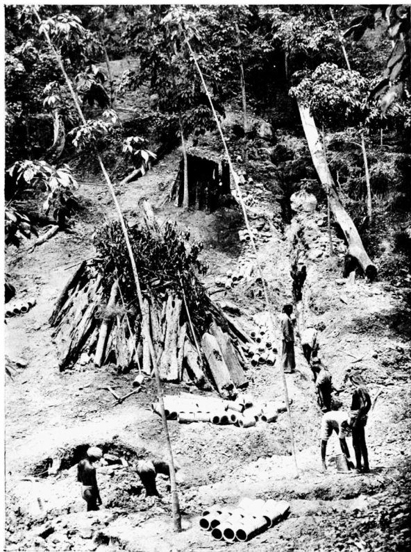
FIG. 3.—BUKIT IJOK ESTATE, FEDERATED MALAY STATES. Subsoil drainage to tap springs on the side of a steep ravine.
