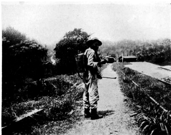
FIG. 23.—ONE OF THE MEN BELONGING TO THE SANITARY DEPARTMENT WITH A KNAPSACK OIL-SPRAYING MACHINE.
