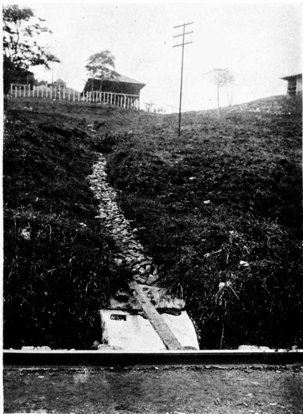
FIG. 13.—A SUBSOIL DRAIN COVERED BY STONES AT ANCON.
